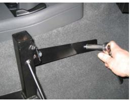
Attach support brace to floor using 1/4" x 1" hex head lag bolts
